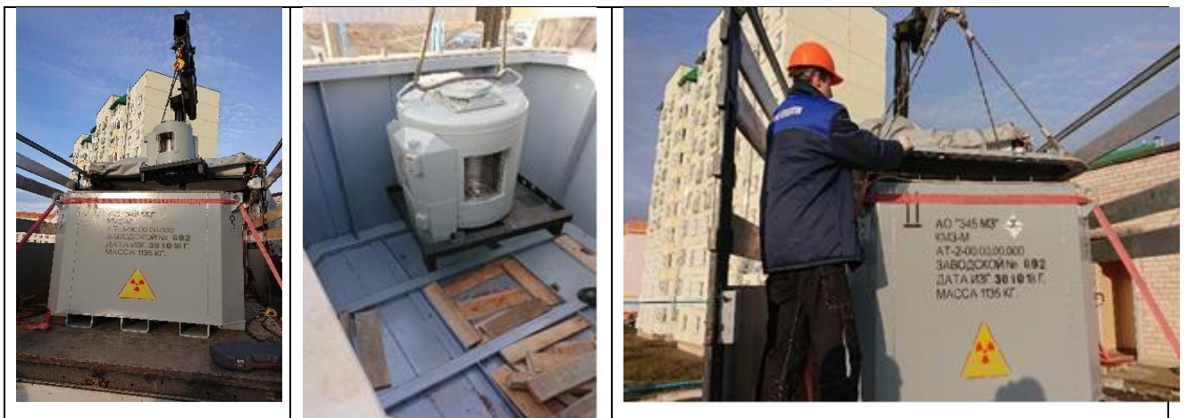
Pic. 19 Loading the radiation head to the KMZ container.
