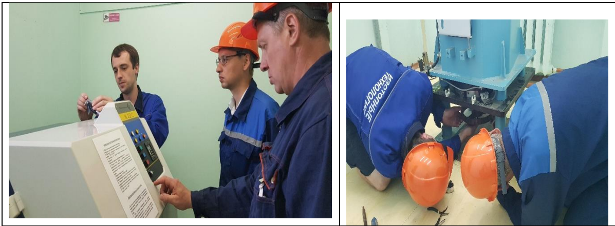
Pic.2 Dismantling the irradiator
