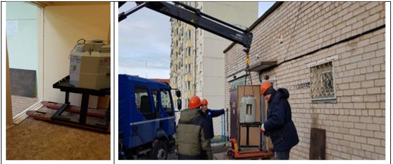
Pic.18 Dismantling of the Gammacell-3000
