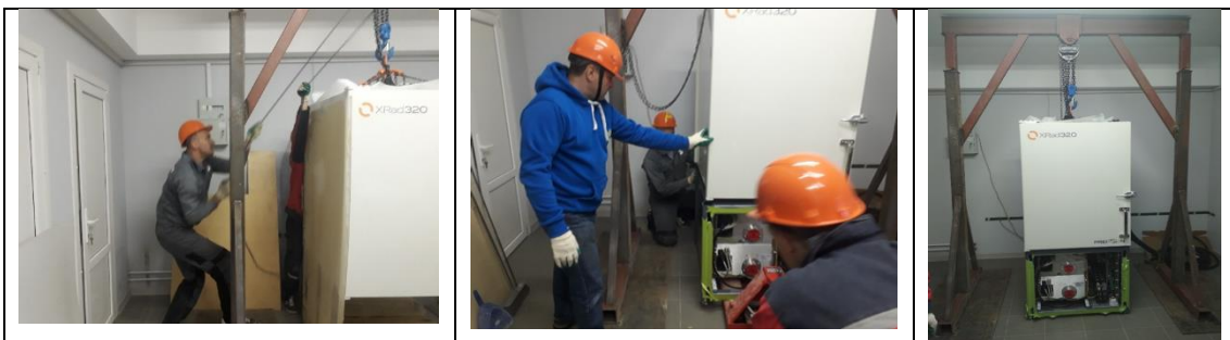
Pic.15 Installation of the X-RAD-320
