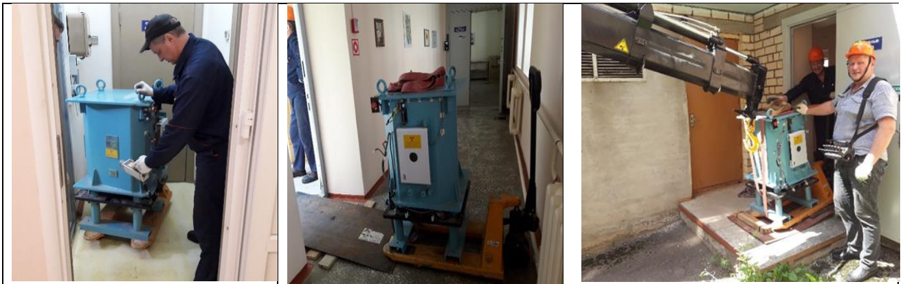
Pic.3 Rigging the radiation head
