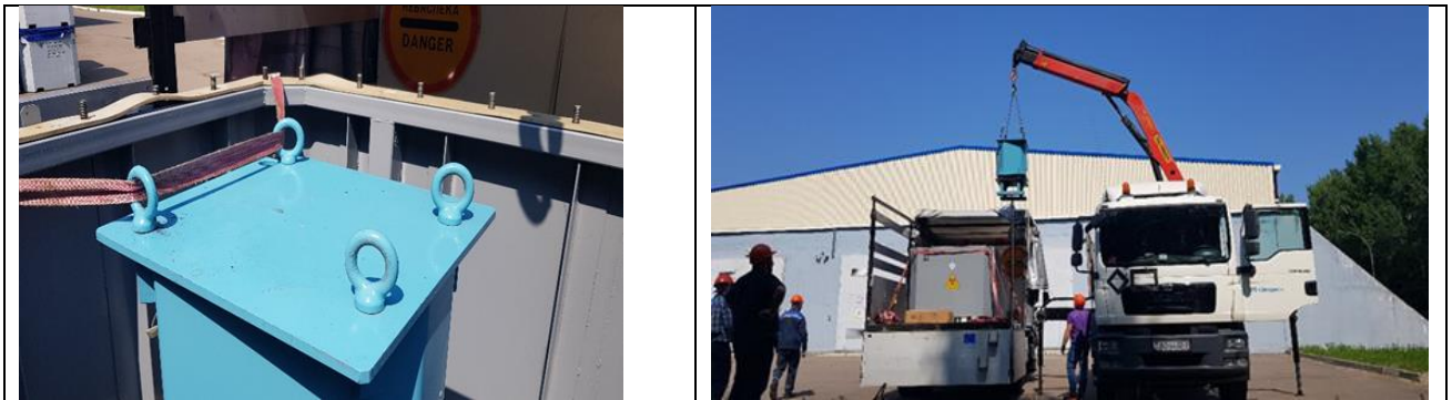
Pic 5. Placing the radiation head with Cs-137 source at the waste disposal facility “EKORES”
